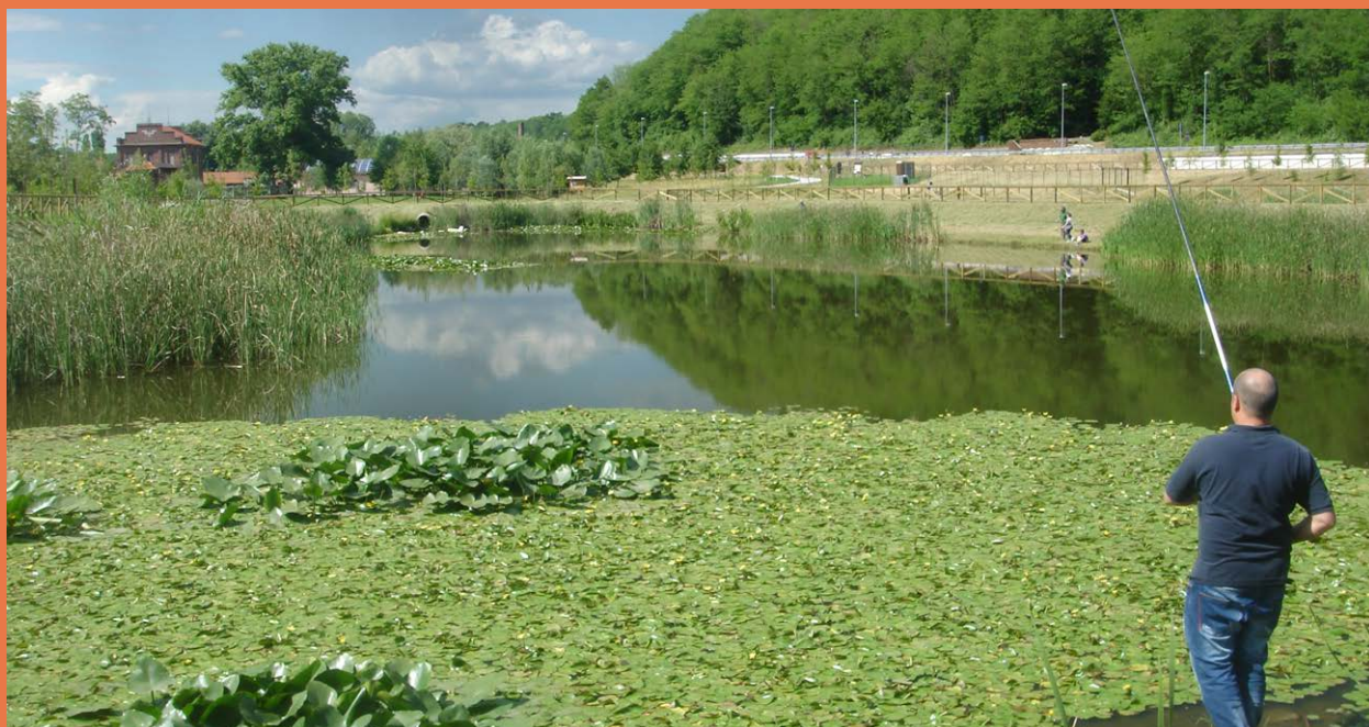
Natural water treatment at Gorla Maggiore water park, Italy. © Nicola Martinuzzi.
